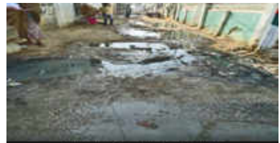
Situation of Lane before construction of sewerage line
