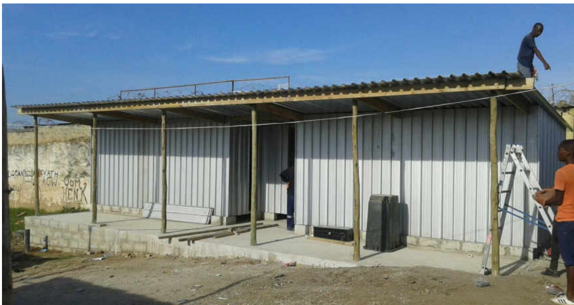
The nearly complete Midrand WaSH Facility.
