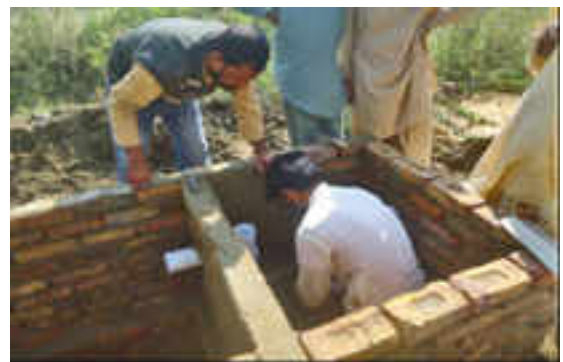
TTBC Providing Technical Guidance (during Construction) to women for T-M (P)
