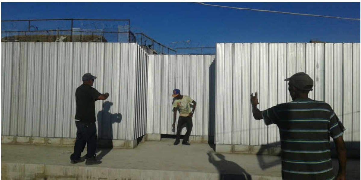
The facility under construction
