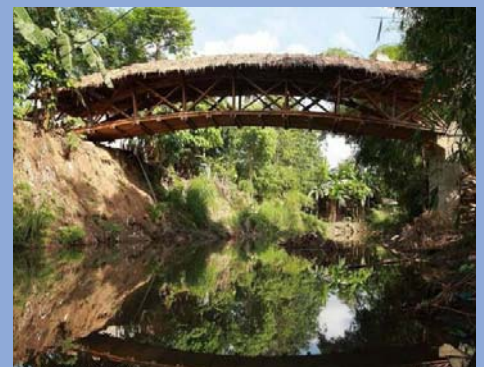
▲ DAVAO : This amazing 23m bamboo bridge provides storm and flood-proof access to three poor communities in the Matina Crossing Federation, who built it with a $7,000 small project loan, and lots of help from some enthusiastic community architects from around Asia.
