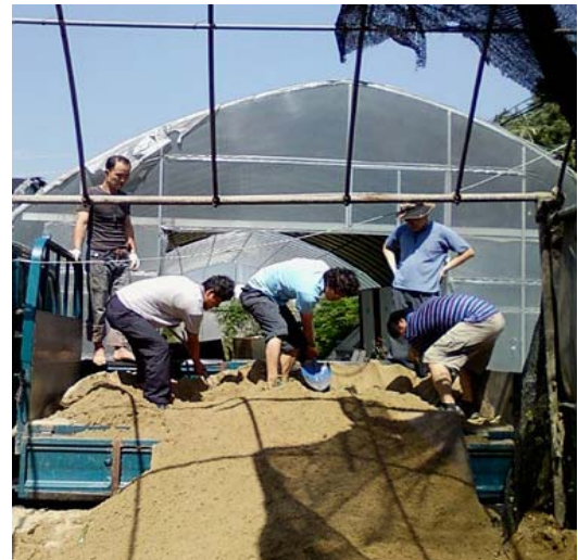
Children's library construction
