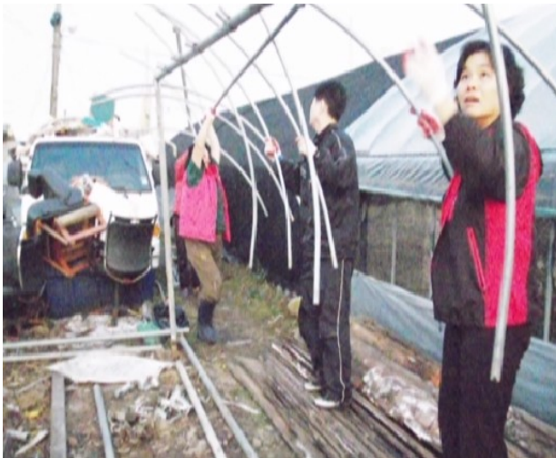
Recycling centre construction
