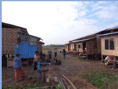
▲ **A new community built in just 3 months** : The people staked out the plots, constructed the infrastructure (with water pumps, toilets, shared septic tanks and simple raised earth lanes) and built the houses themselves, in sub-groups, very simply and well. They figure that these simple houses will last about 7 years, when they'll be better-off and be able to upgrade them.
