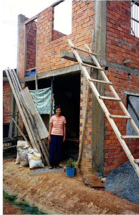
A lot of the families didn't want to take very big loans, so they built incrementally, starting with a sturdy concrete frame and finishing later.
