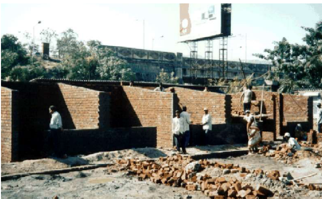
Construction of the one-story row-houses at the Kanjurmarg transit camp begins, according to the layout plans the people developed themselves.
