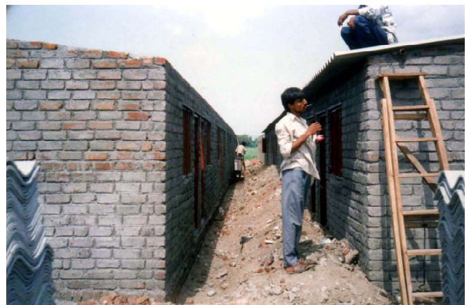
The construction was done by a local contractor, but the railway community members supervised the construction and purchased all the materials.
