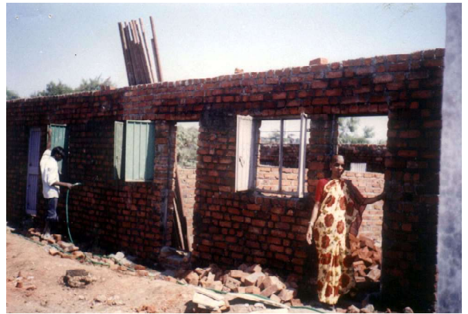
There's Banoo, one of the senior Mahila Milan leaders, visiting the construction site to help out with various tasks in Kanjurmarg.
