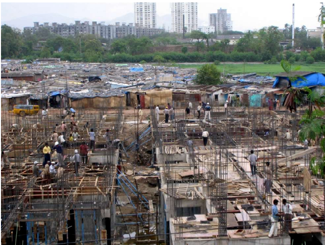
▲ The permanent SRA housing blocks being constructed, in the foreground, with the remains of the Kanjurmarg transit housing in the back.
