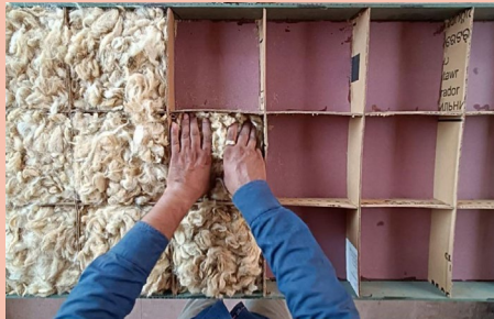
Sheep wool sourced locally is prepared and assembled into roof insulation, linking cooling solutions with local livelihoods.
