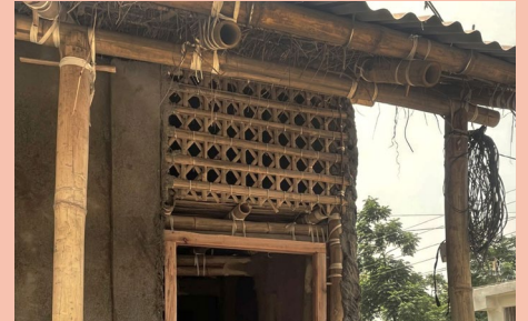
Above, traditional bamboo lattice allows air movement while filtering light and visibility. Below, the upgraded design mirrors traditional patterns while strengthening durability.
