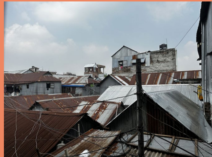
Clusters of tin-sheet houses in Dhaka absorb and radiate heat throughout the day, turning entire neighborhoods into heat traps where both indoor and outdoor spaces remain uncomfortably warm well into the evening.
