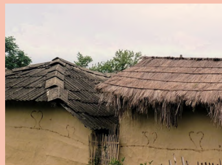
In Nepal, thatch is placed over cement tiles or iron sheet roofs to keep rooms cooler.
