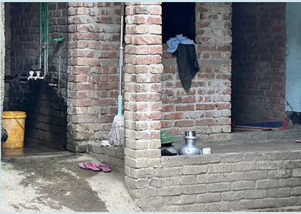
Sprinkled water on floors and walls.
