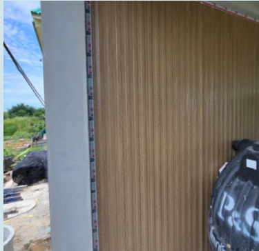
Insulated metal sheet "sandwiches" as walls.
