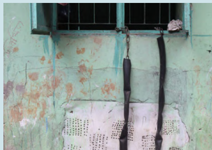
Perforations under cooking areas to release air.
