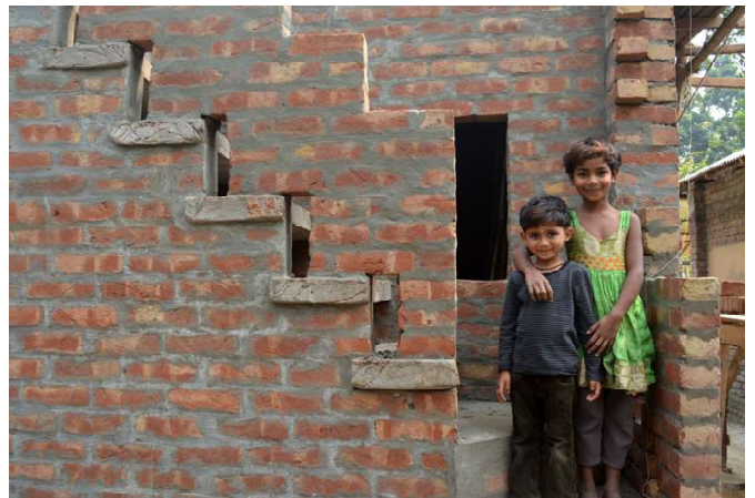
The houses incorporated several cost-saving building techniques that had been popularized decades earlier in India by the architect Laurie Baker. One of those techniques is this stairway made from pre-cast and reinforced stair slabs.
