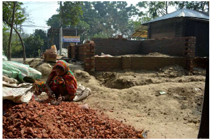
Here the brick masonry walls of the first model house are starting to go up. All the unskilled labor was provided by community members.
