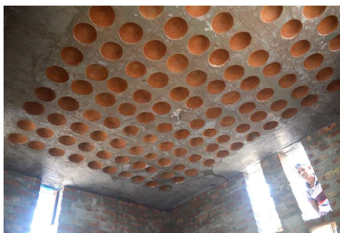
Another cost-saving building technique from Laurie Baker was the "filler slab", in which the use of expensive concrete in floor slabs is much reduced by placing terra-cotta pots in the formwork, to create voids where the material is not doing any structural work.
