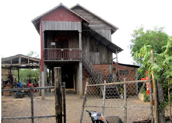
Ten years later: the lower part of this house has been partly enclosed, and a bathroom and cattle shed have been added to the sides.
