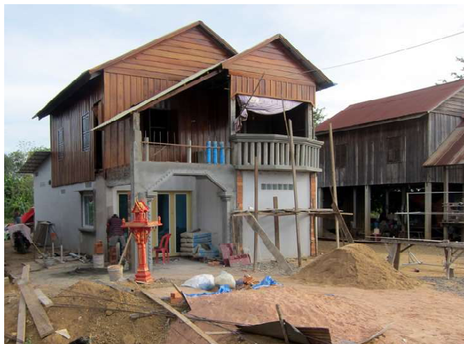
The lower part of this house is in the process of getting a deluxe upgrading, with a full masonry-enclosed ground floor and addition at the back.
