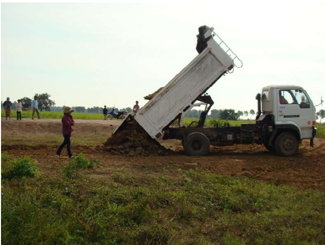
The municipal government paid to have earth brought in to fill the land for the access and internal roads, and part of the housing site.
