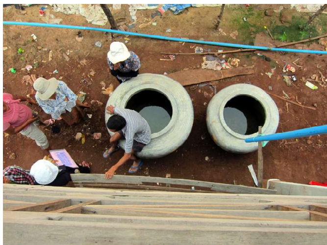
Traditional Khmer houses are always designed to catch the rain during the monsoon season and channel it into big pots around the house, which provide water for drinking and washing in the dry season. The houses in the new project are keeping alive this time-tested solution.
