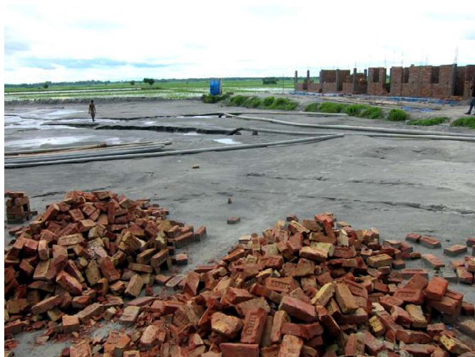
Some photos from the Mandartola site in July 2013, when almost half the 236 houses were either finished or well underway. The land-filling (above right) also continued, using the piped-in liquid sand system, which is a common landfilling technique in Bangladesh.
