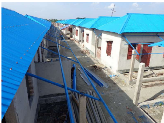
The galvanized iron roofing sheets are painted blue on the outside to reflect the fierce Bangladeshi sun, and white on the inside.
