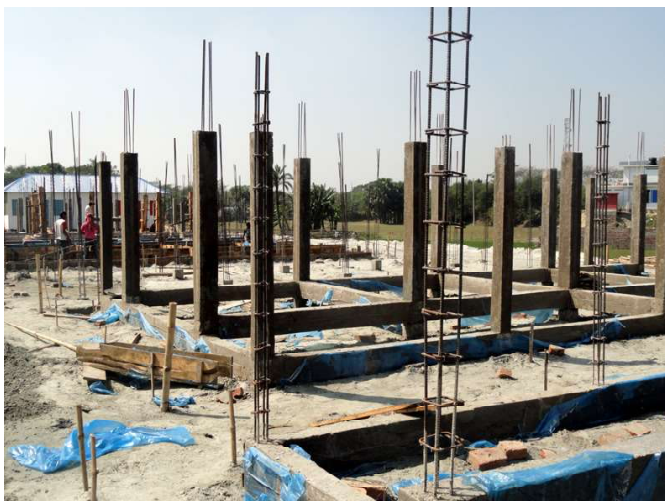
The CDMP's standard disaster-resilient house was built very sturdily, on a three-foot plinth, with bricks and steel-reinforced concrete frames. The finished house cost US$ 3,000 to build.
