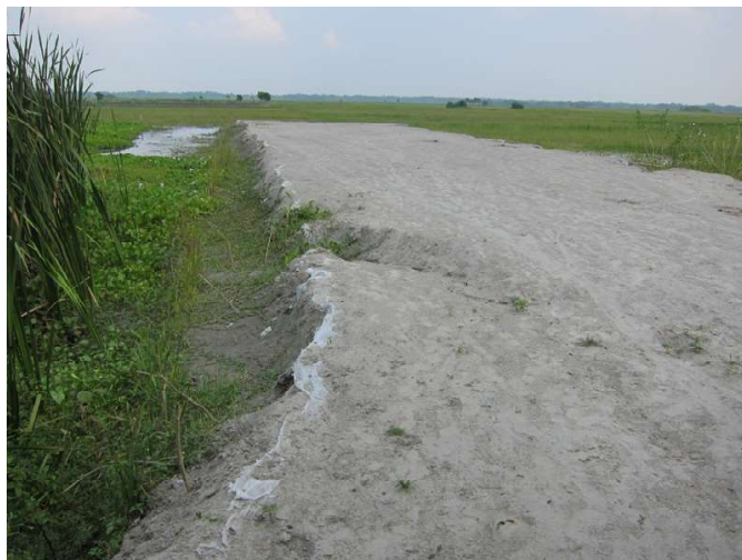
The low-lying rice paddy land had to be filled by almost six meters, to above "historic flood levels" before construction work could begin.
