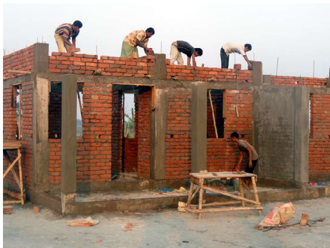
The CDMP's standard disaster-resilient house was built very sturdily, on a three-foot plinth, with bricks and steel-reinforced concrete frames. The finished house cost US$ 3,000 to build.
