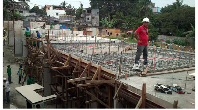
9 Here the formwork and steel reinforcing is being prepared so the concrete can be poured to make the floor slab for the second floor units.
