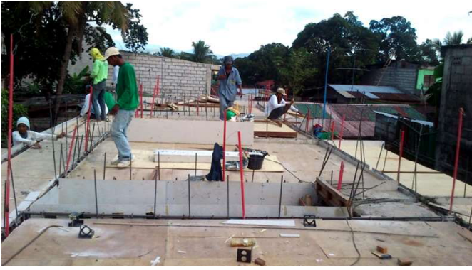
8 This "Plaswall" construction system is something like building a house out of cards - but very strong and heavily-reinforced cards.
