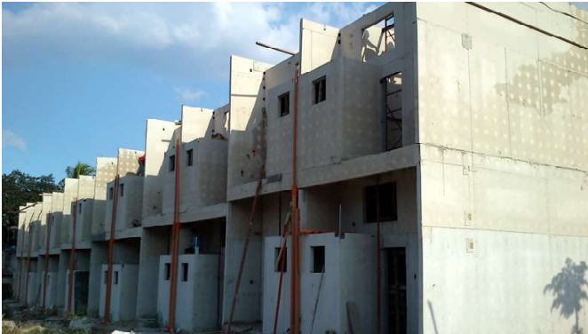
10 Here the construction of the walls and floor slabs for both first and second floor units has been completed and is ready for the roofing.
