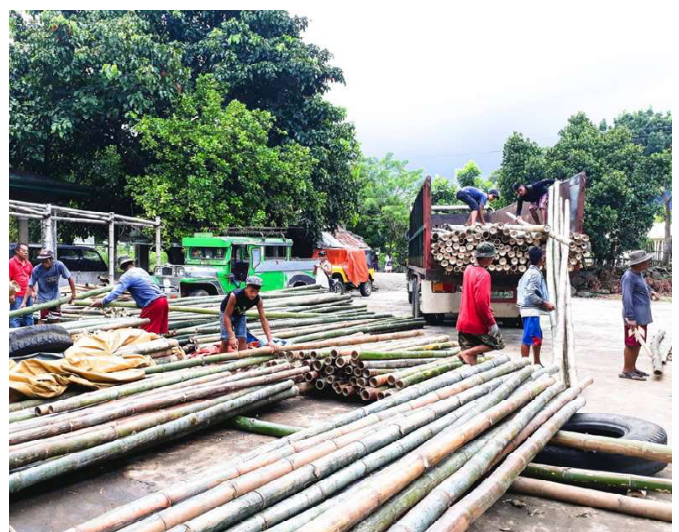
Unloading the treated bamboo poles, which became the main structural material in the new houses in the Ati community.
