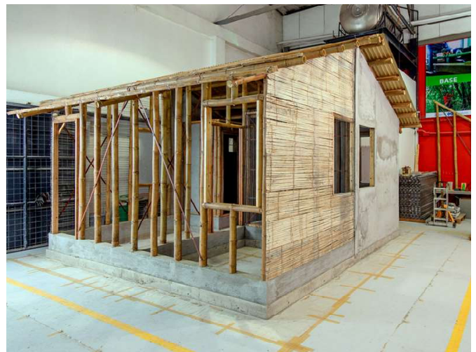
The Base Bahay Foundation has built this full-size model of a house built using their cement bamboo technology, to show how it works.
