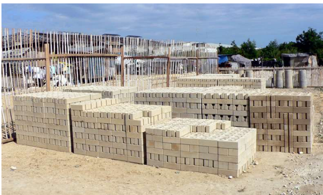
Here the blocks are stacked after curing, ready to be used. Each rowhouse required 2,500 blocks, and making them was quite a job.
