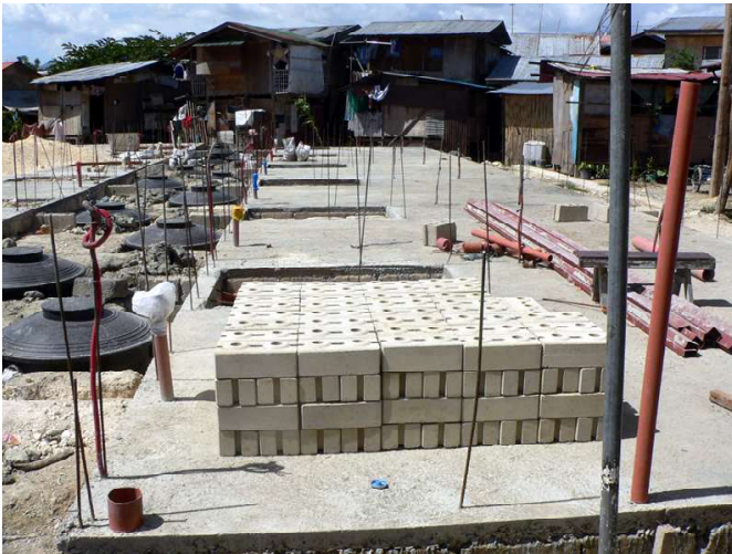
The CEB blocks are load-bearing, so there isn't any need for expensive reinforced concrete frames. That made the construction much cheaper, simpler and faster. The blocks are reinforced with a little steel and cement, as can be seen in the photo above (right).
