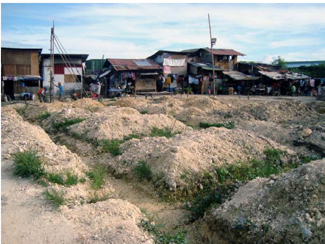
Here the trenches for one row of houses have been dug and are ready for the construction of the foundations to begin.
