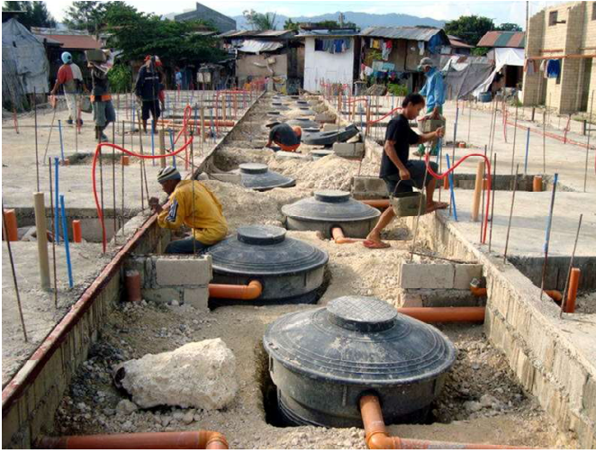
These are the Kotek septic tanks which the community people opted to use, at the back of the houses. Each tank serves four houses.
