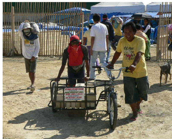
Some clever fabricator rigged up this cart for carrying the CEB blocks to the construction site, which was a few hundred meters away.
