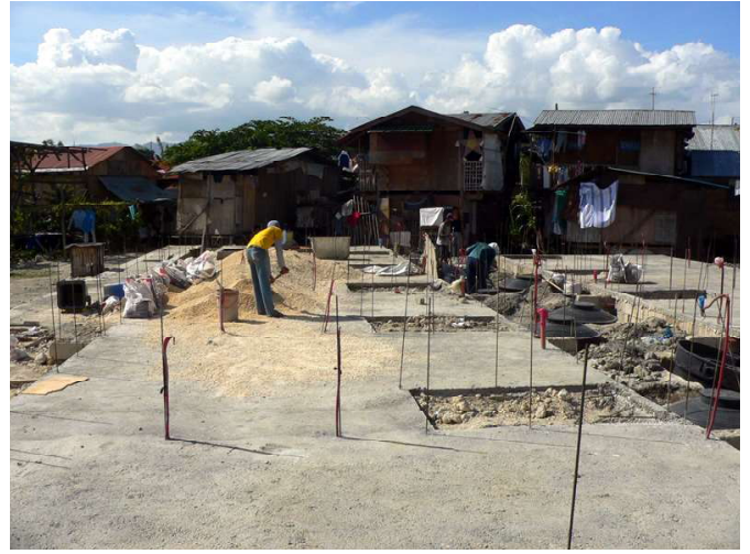
Here the foundation and plinth of a row of houses is finished and ready for the construction of the walls to begin.
