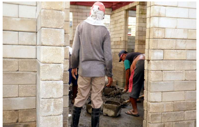
Building the walls with CEB blocks: The blocks have a natural golden color, which comes from the local soil in Mandaue, and they are hard enough and durable enough that they don't have to be plastered or painted, inside or out. They do have to be protected from water though.
