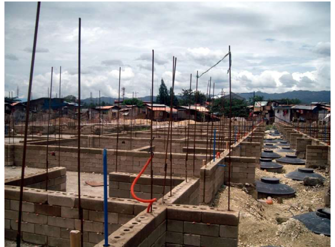
The CEB blocks are load-bearing, so there isn't any need for expensive reinforced concrete frames. That made the construction much cheaper, simpler and faster. The blocks are reinforced with a little steel and cement, as can be seen in the photo above (right).
