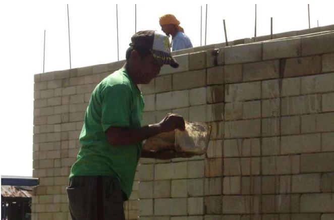
Building the walls with CEB blocks: The blocks have a natural golden color, which comes from the local soil in Mandaue, and they are hard enough and durable enough that they don't have to be plastered or painted, inside or out. They do have to be protected from water though.
