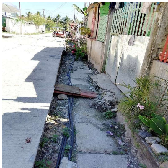
The municipal roads that go through the Los Amigos resettlement site are higher than the lots, and that has caused flooding problems.
