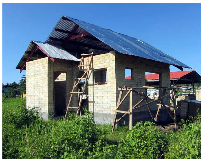
Here are two photos of the first demonstration "core house" that was built on the Los Amigo site: the front side (on the left) and the back (on the right). The house was designed to be only partly finished, with one big room inside, a toilet out back, and a sturdy roof of corrugated iron sheets.
