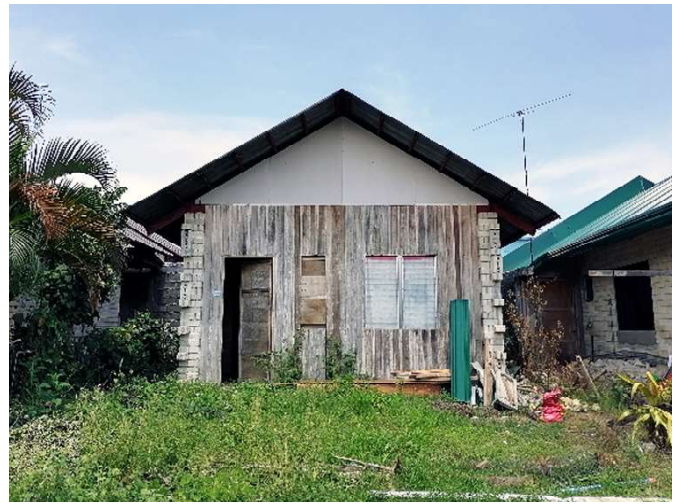
Here is one of the original "core houses", with the front wall built of light materials, with a window and a door, ready for expanding the house to the front later on, when the resources are available.
