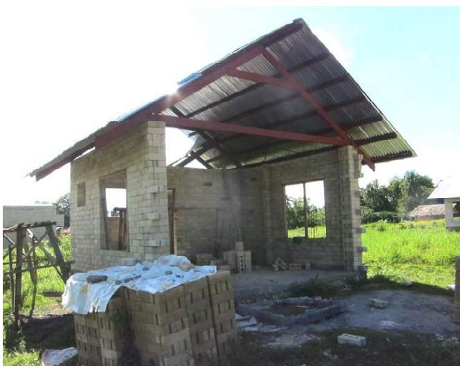
Here are two photos of the first demonstration "core house" that was built on the Los Amigo site: the front side (on the left) and the back (on the right). The house was designed to be only partly finished, with one big room inside, a toilet out back, and a sturdy roof of corrugated iron sheets.
