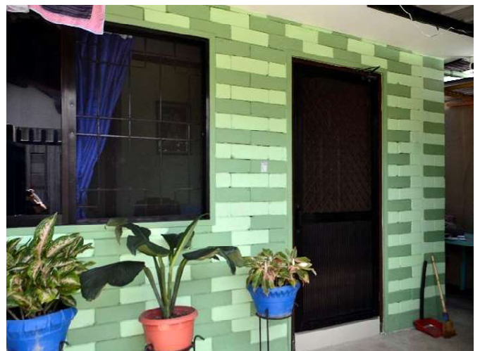
This family has replaced the front wall with ICEB blocks and aluminum windows and doors, and painted the blocks bright green.
