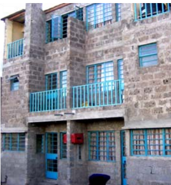
▲ The Kenya federation's housing project at Kambimoto was one of the first in Africa to show a densely-packed housing solution with 2 and 3-story houses.
