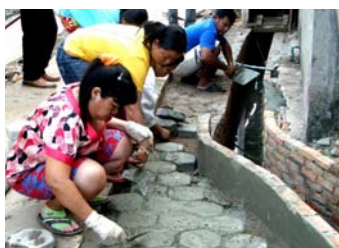
Lao's first on-site slum upgrading project, at Nong Duang Thung in Vientiane.
