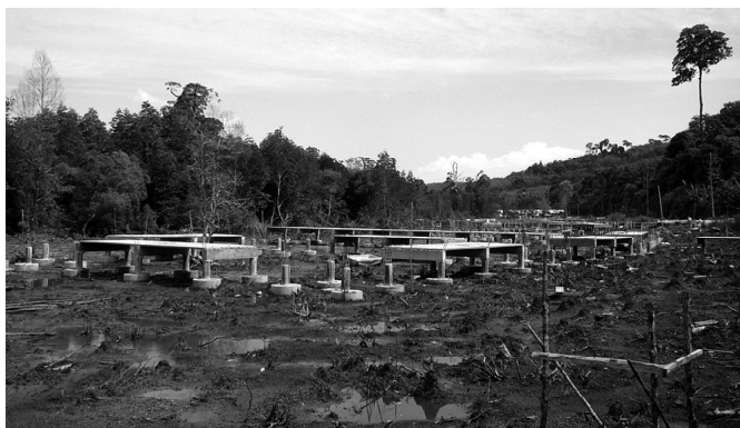
This is a photo of the new site when the system of "floating" concrete community walkways was almost finished.
