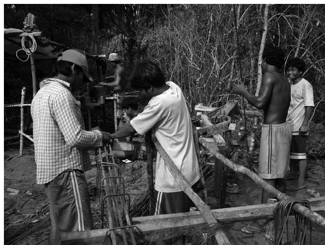
The columns had to be extra strong to withstand future tsunamis, so there was training in how to build them to a higher than normal standard.
