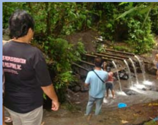
The gravity-flow water supply system which the Masawarag community in Albay is building, with bamboo pipes.
