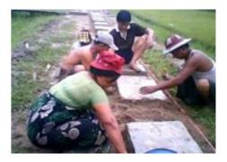
**Home-made paving slabs:** The land in the third project is low-lying and prone to floods, so paved pathways became essential. There wasn't enough budget for concrete paving, though, so the community people cast their own simple cement paving slabs and set them in raised beds of sand. It cost only \$500 to make pathways this way throughout the whole community.
