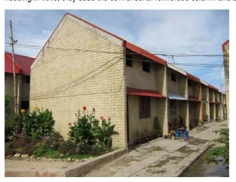
purchased in the market. After constructing the first batch of houses using the load-bearing compressed earth blocks at LTHAI they find that the construction is 30% cheaper. Why? They eliminate the need for plastering inside and out, the system uses less steel and less cement. Plus, with the load-bearing block system, they can go up to 4 stories, but just have to arrange 4 blocks at the corners to make an internal columns.
