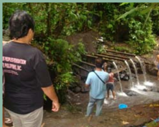
The gravity-flow water supply system which the Masawarag community in Albay is building, with bamboo pipes.
