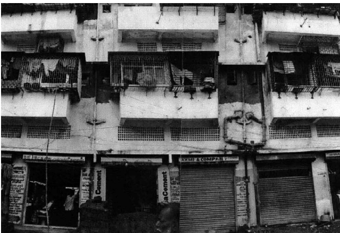
Here coop members follow the long Mumbai tradition of putting up grilles and awnings around balconies, to let the air in and keep the rain out, but make room for hanging out the wash to dry.
