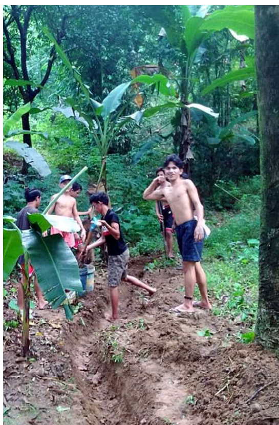
In this photo, some of the boys in the community are helping to dig trenches, as part of a project to upgrade the water supply system.
