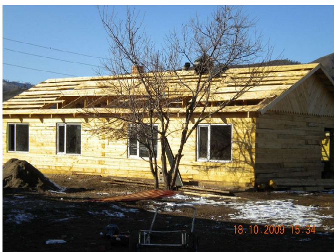
The heavy timber built houses almost ready for the roofing and siding to be put on.
