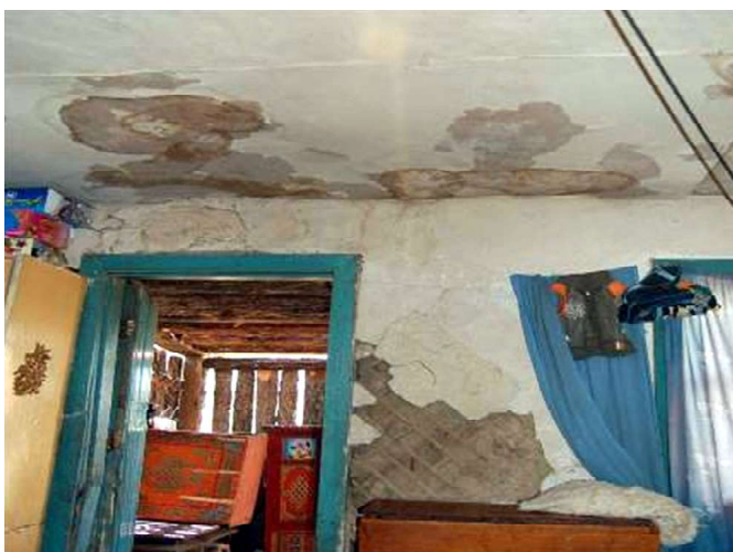
Inside conditions before the project, with water leaking in through the roof, crumbling walls and lack of insulation for the fierce winters. e time for all good men.
