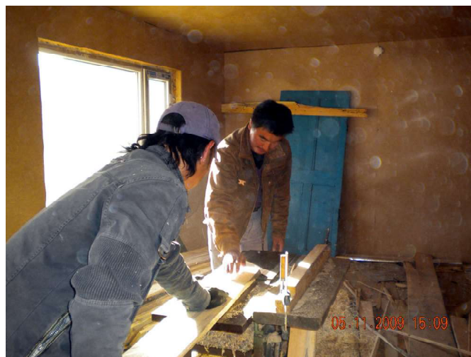
Work on the houses inside, with the double-glazed windows in the background, which reduce heat loss and cold penetration.
