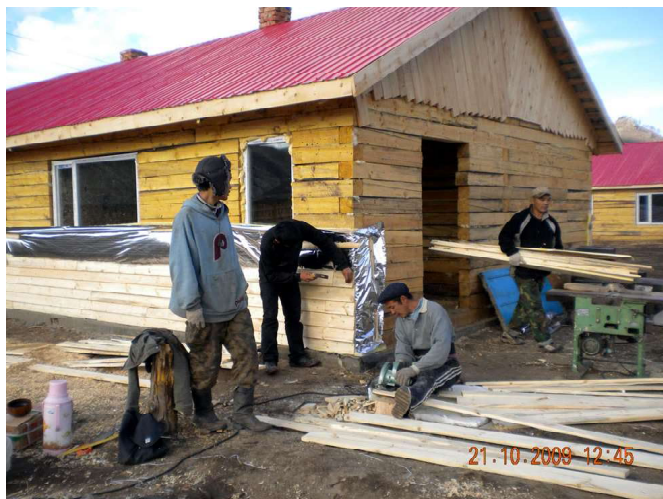
Construction of the new houses underway. with residents themselves providing all the carpentry skills. Note the heavy log walls.
