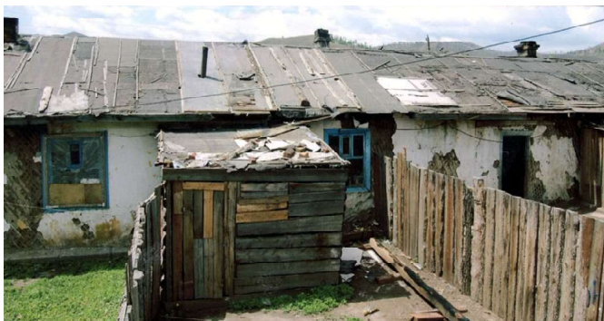
Housing conditions before the rebuilding, with leaky roofs, deteriorating mud plaster walls and uninspiring privies.
