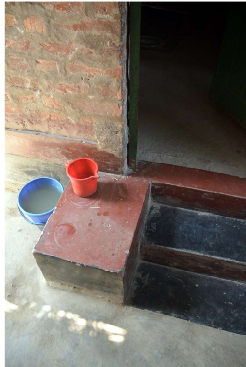
In this photo you can see the flush-pointing of the brick work, which makes the wall nice and smooth, without having to fully plaster it.
