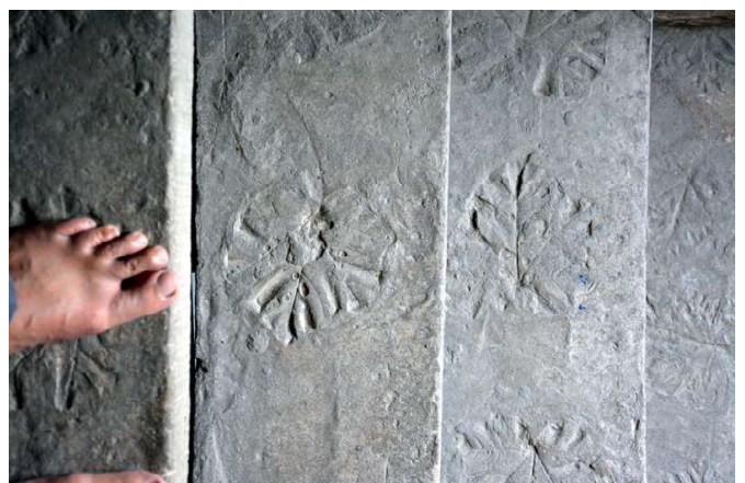
Just for fun, some of the pre-cast stair slabs were ornamented with the impressions of leaves pressed into the wet concrete.
